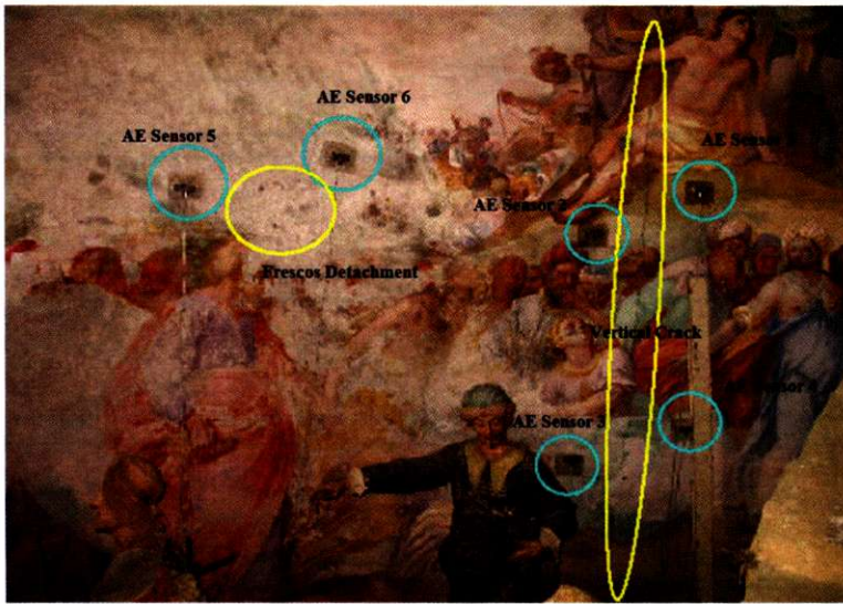
Fig. 17.3 Chapel XVII: view of the monitored damages and position of the AE sensors
